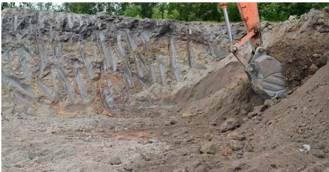
Figure 1: Stage 1 mining of extensive graphite mineralization at surface.
