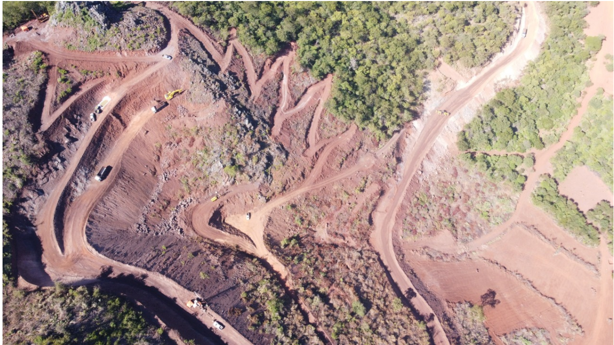
Figure 2: Mine Access & Road Infrastructure
