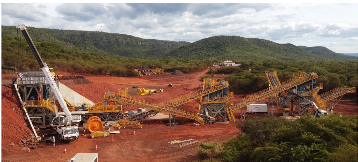
Figure 3: Crushing & Screening Plant assembly in progress
