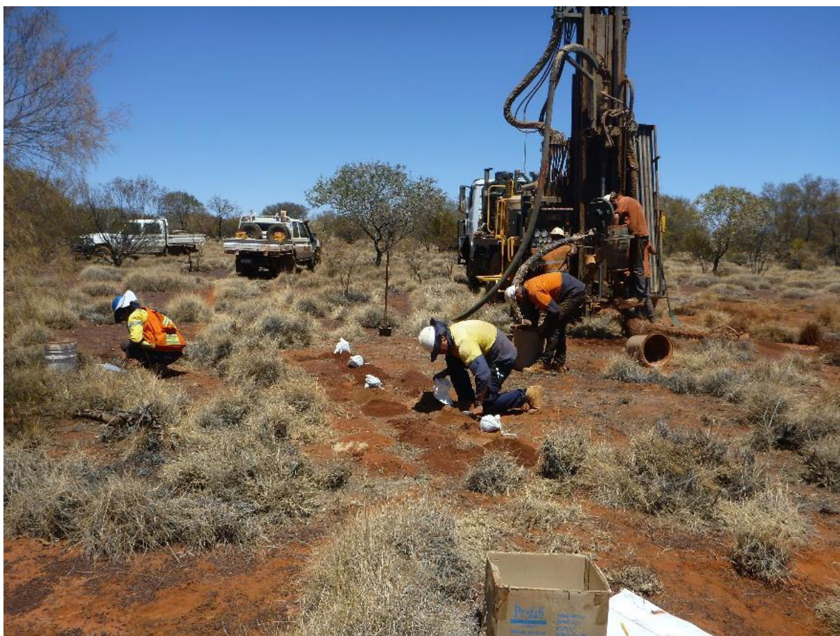
Figure 13 - Drilling at the Grimlock Prospect on the Lake Mackay JV, October 2020.
