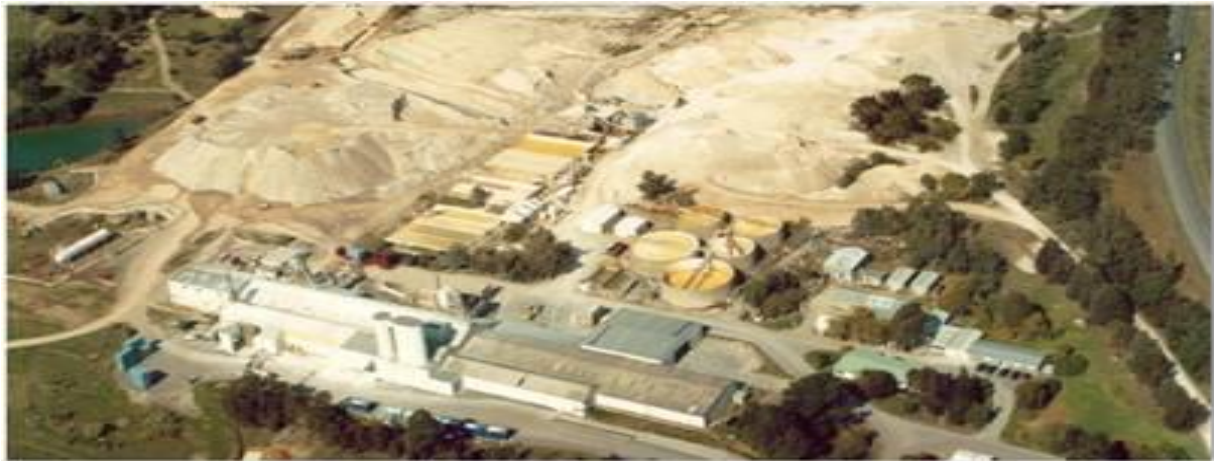
Pittong processing plant facilities
