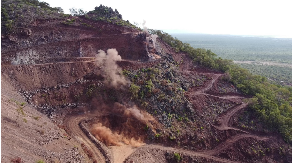
Figure 2: Tombador Project First Blast
