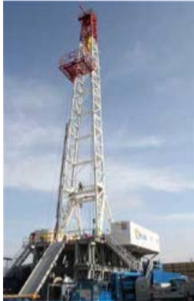
Graham Drilling Rig 5
