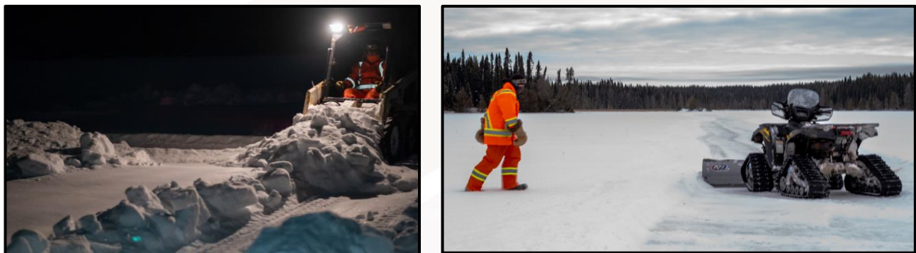
Figure 6 – Winter Drill pad preparation on the frozen lake at the Kasagiminnis Gold Deposit
