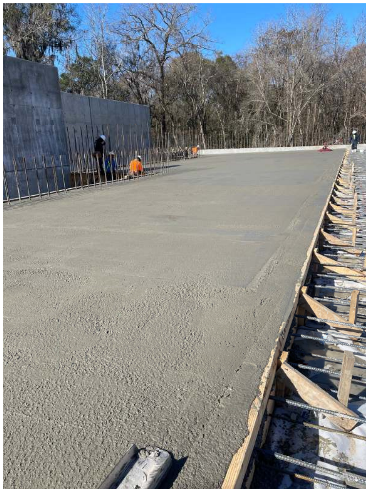
Figure 3. EdenCrete® enhanced concrete slab being installed
