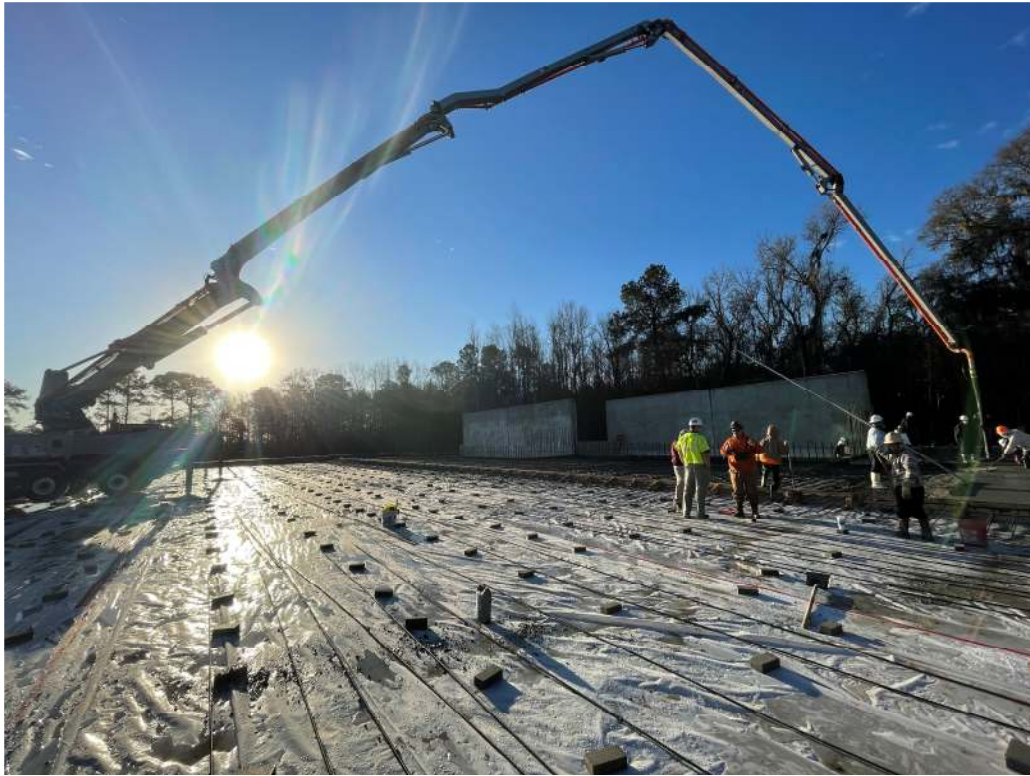
Figure 2. EdenCrete® enhanced concrete slab being installed
