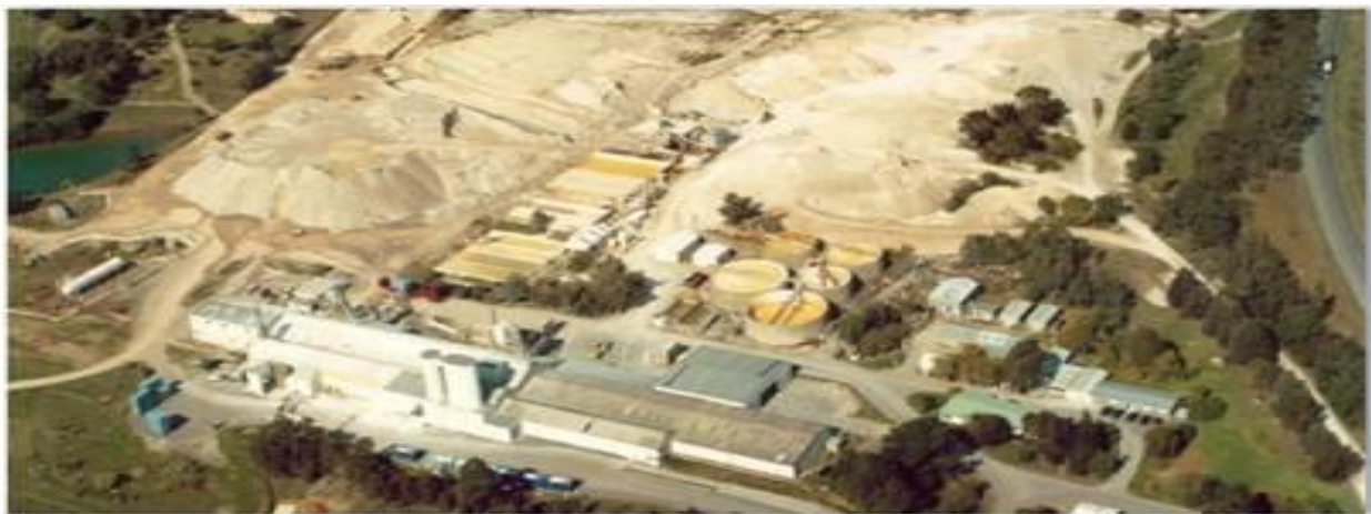
Pittong processing plant facilities
