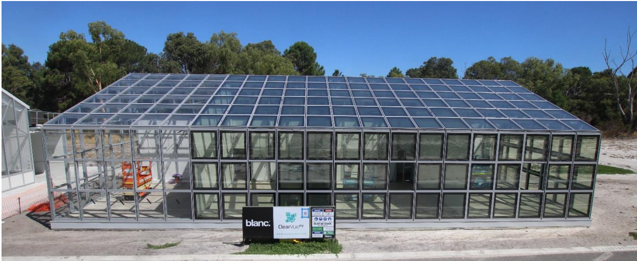
Three versions of ClearVue's PV glazing installed onto rooms 2,3 and 4 of ClearVue's solar greenhouse at Murdoch University, Western Australia. Room 1—a trial 'control' room (far left) showing single pane glazing only.
