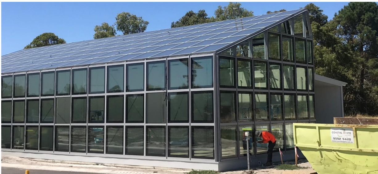
Three versions of ClearVue's PV glazing installed onto rooms 2,3 and 4 of ClearVue's solar greenhouse at Murdoch University, Western Australia. Room 1—a trial 'control' room (far left) showing single pane glazing only.
