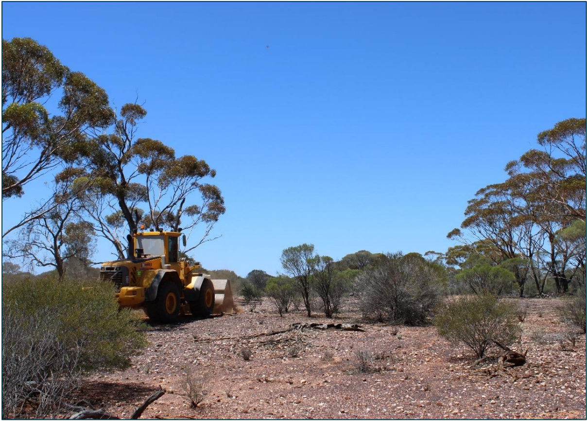
Figure 3: Loader clearing AC lines for drill rig access.
