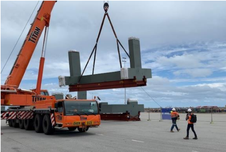
Offloading headframe and winder at Henderson Port
