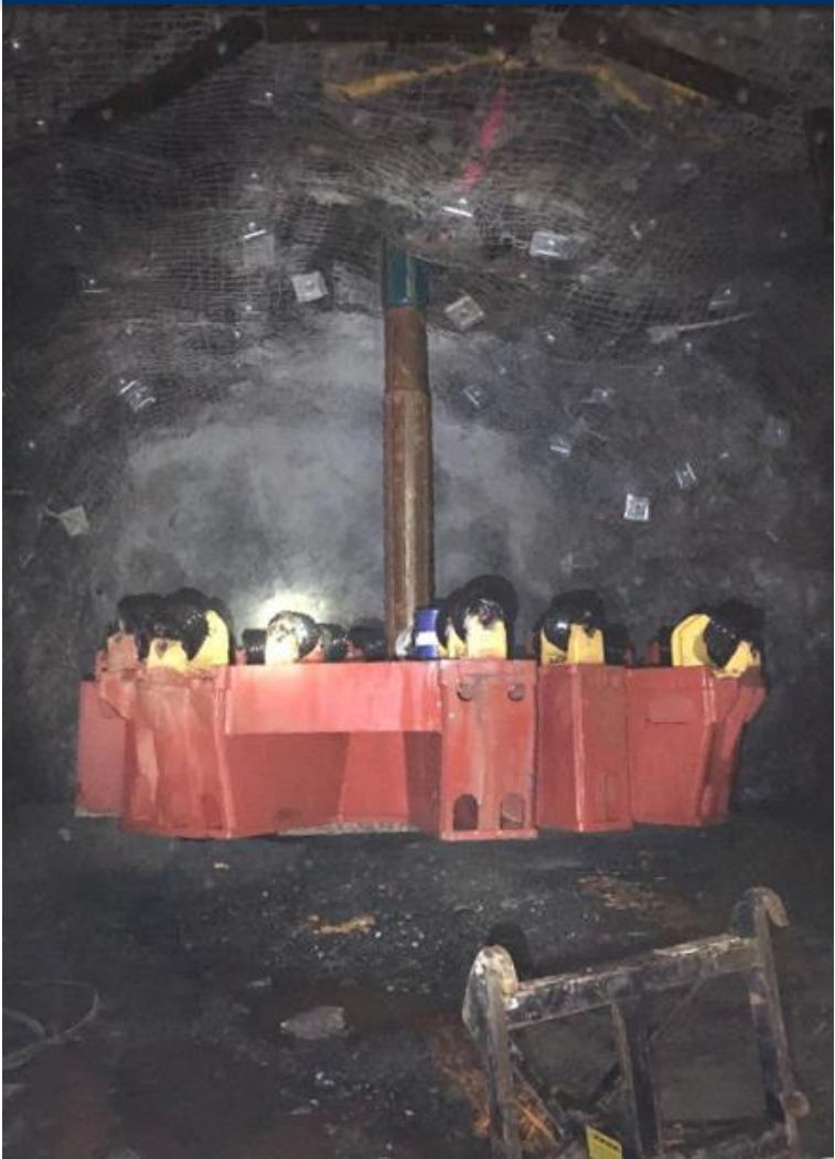
Reaming Leg 1 of the 5.7m diameter production shaft
