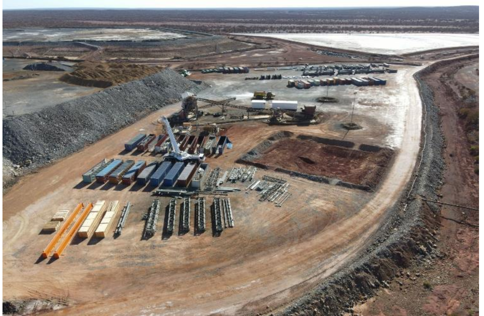
Cosmos laydown yard with headframe and winder components ready for construction
