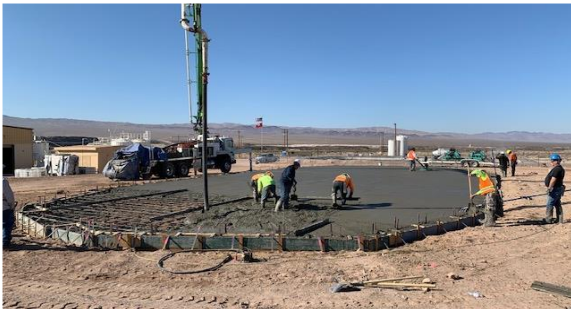
Figure 4 | Photo showing concrete pour for materials warehouse
