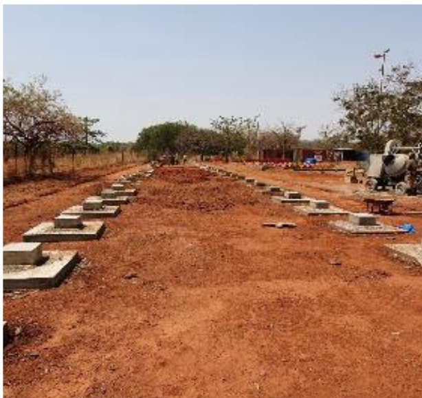
Foundations for temporary power plant
