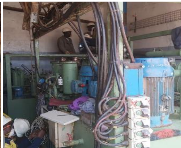
Lubrication system replacement
