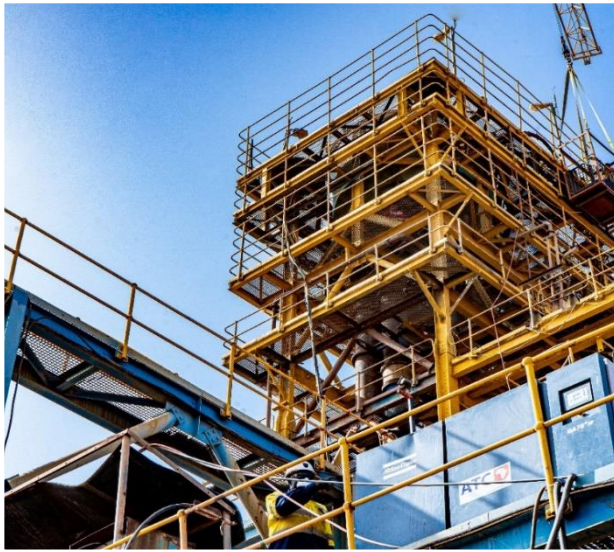
Structural steel replacement, blasting and painting
