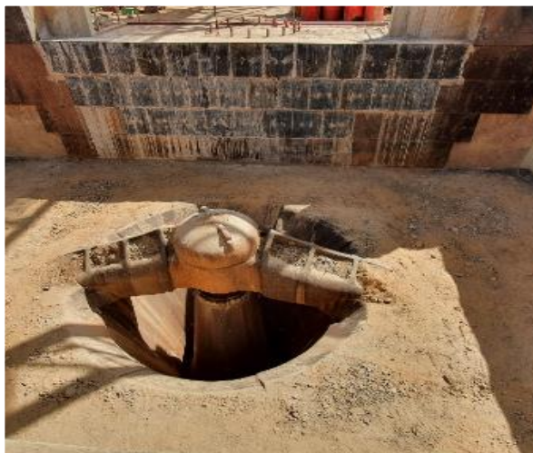
Primary crusher dump pocket liner replacement
