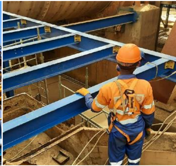
Mill structure steel replacement
