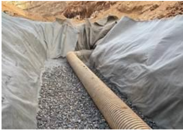
Tailings dam drainage upgrade
