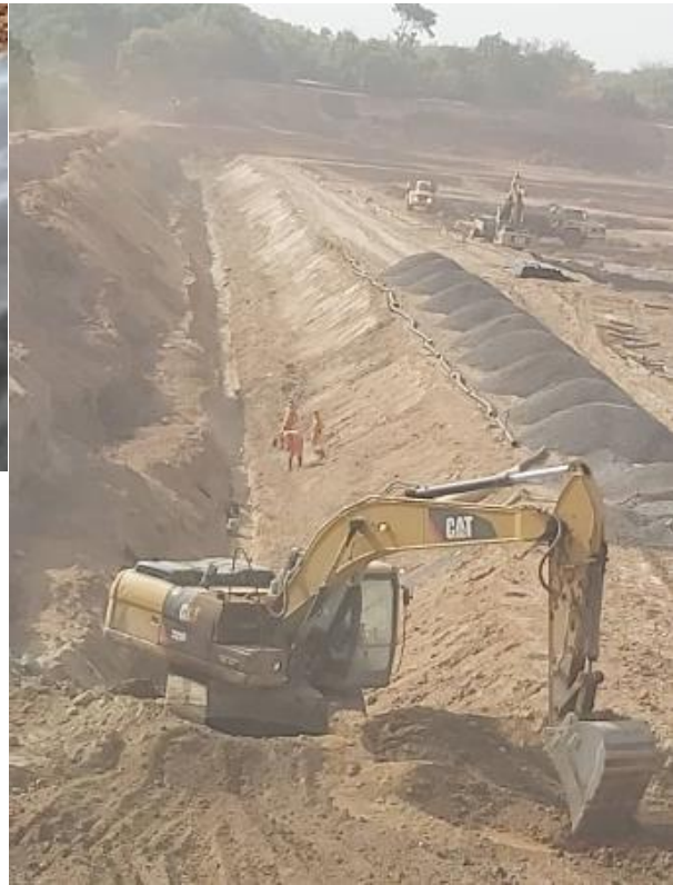
Tailings dam drainage upgrade
