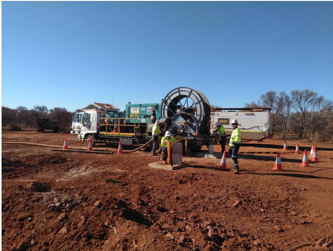
Figure 6: Water Production Bore Pump Testing
