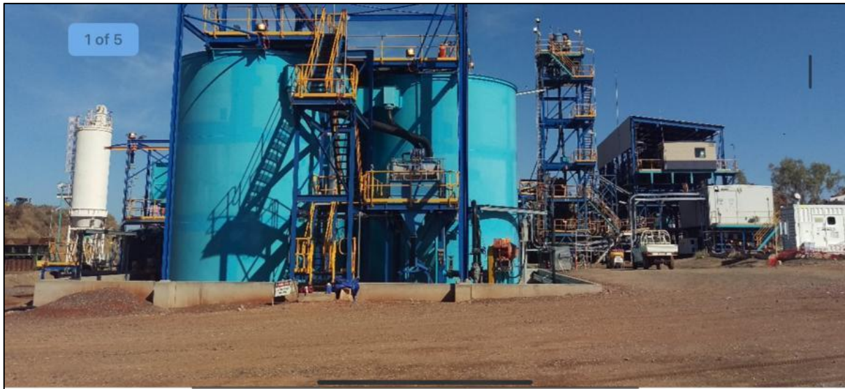
Figure 14: Round Oak Minerals Pty Ltd (ROM) CIP plant located in Cloncurry. All Golden Mile ore under the JV agreement between ROM and Ausmex must be processed at this plant.
