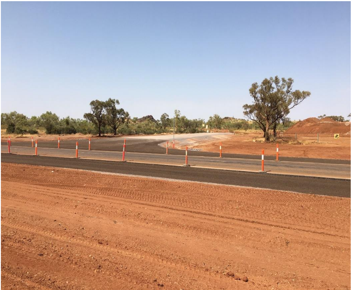
Figure 8: Recently completed Mt Freda Haul Road & regulatory highway merging intersection.
