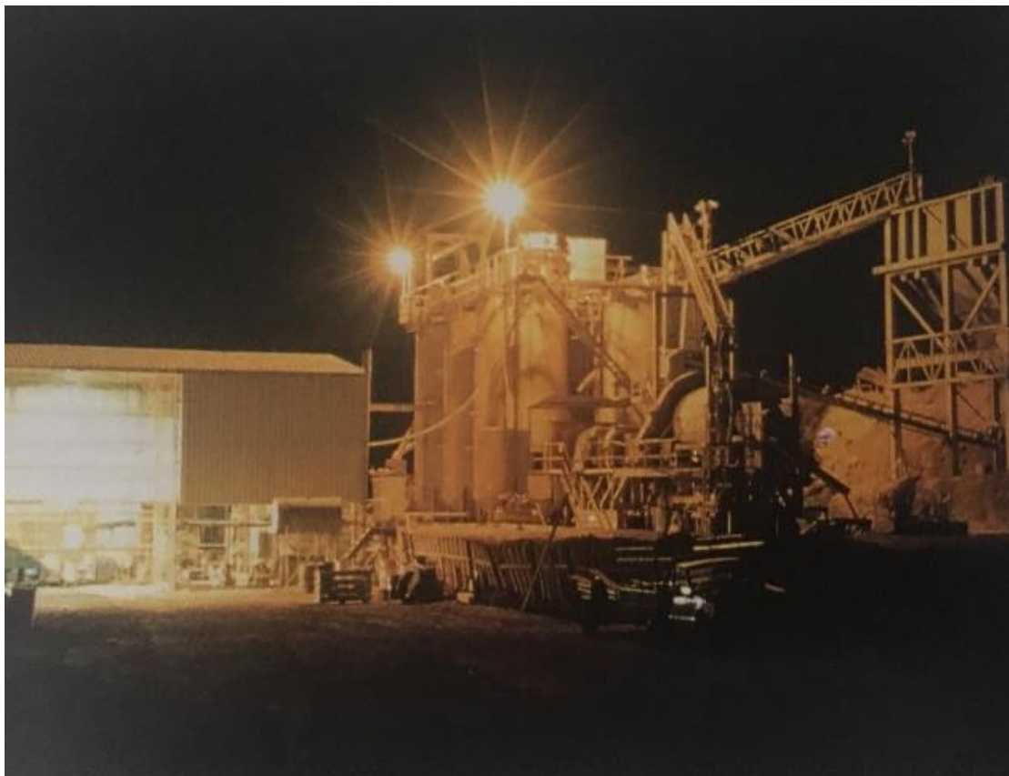
Figure 4: Mt Freda 24-hour operational Gold CIP processing plant late 1980's.
