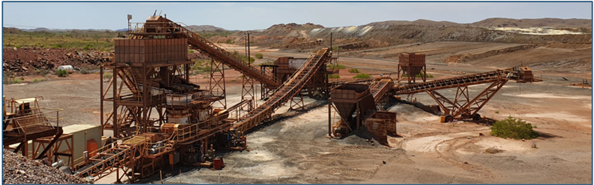
Figure 3: Crushing plant to be refurbished and upgraded to include smart sorting machines.
