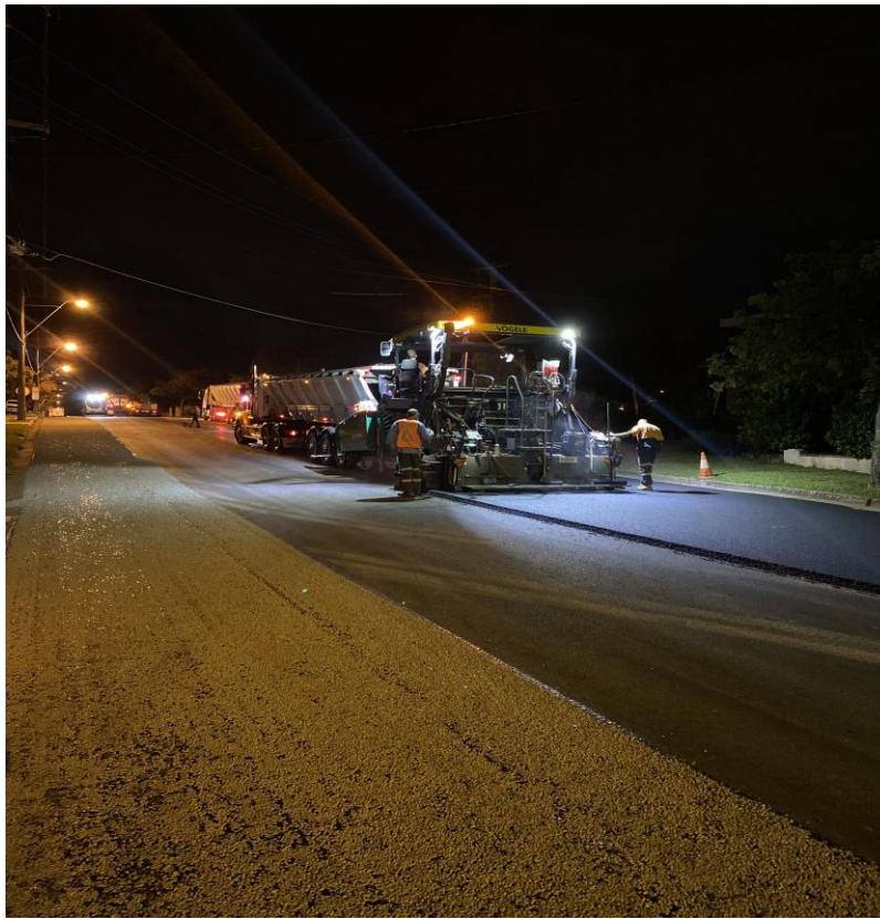
Zero Road Asphalt being laid at King Street, Moreton Bay January 2021 (Source: Ausee Asphalt Pty Ltd)
