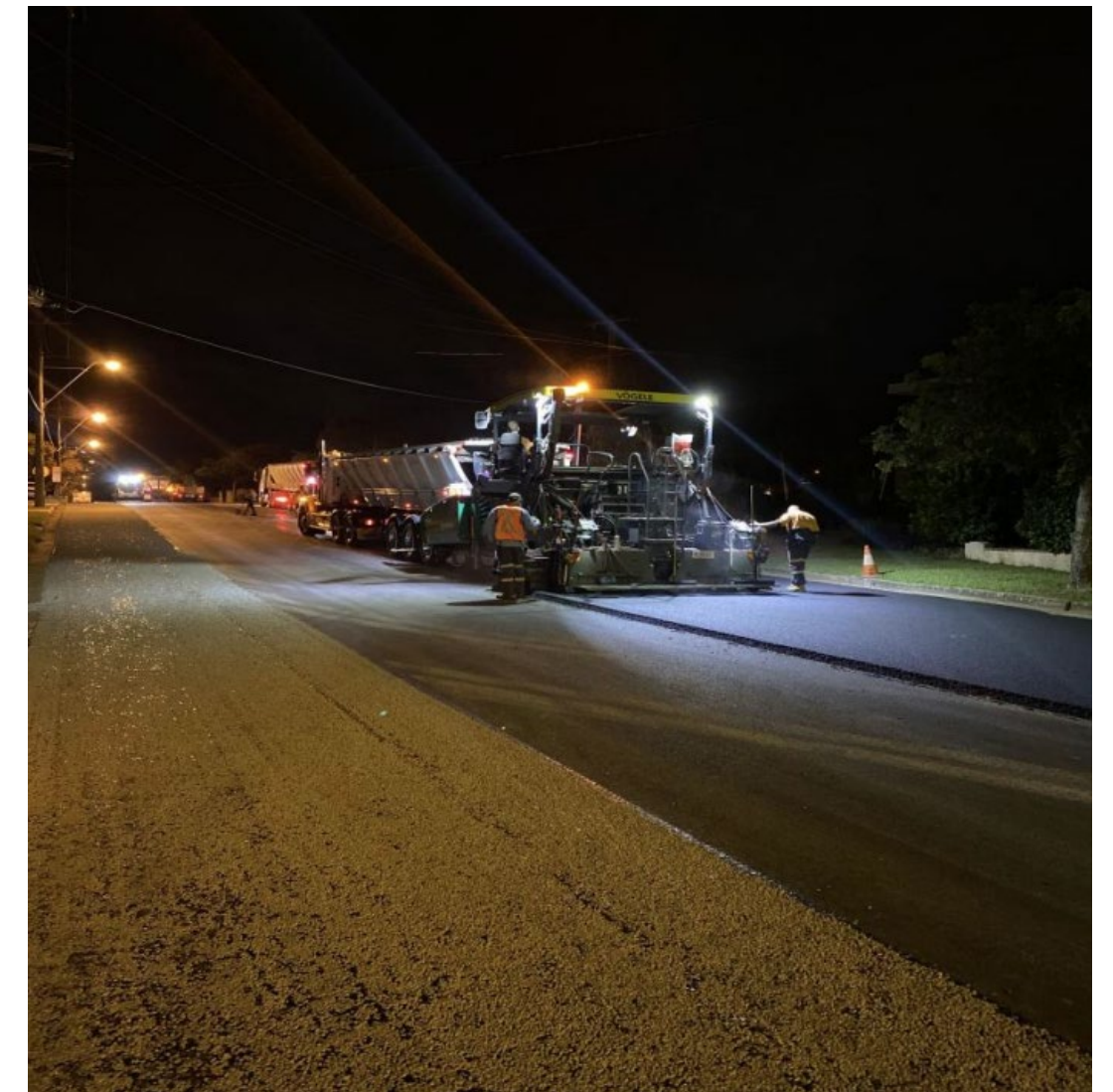
Zeroad asphalt being laid at King Street, Moreton Bay, January 2021 (Source: Aussee Asphalt Pty Ltd)
