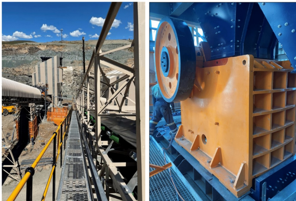
Installation of by-pass conveyor (left) and primary jaw crusher (right)
