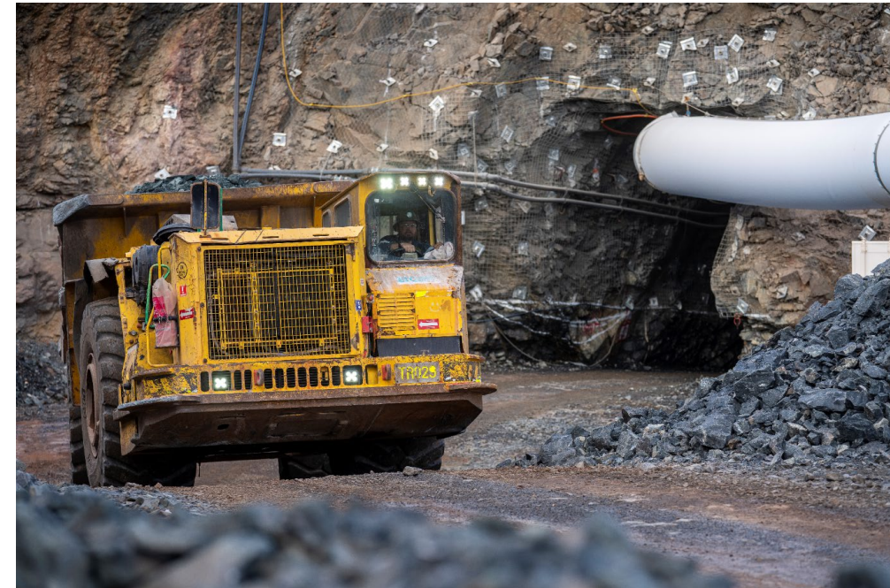
Underground portal works commenced in September 2020
