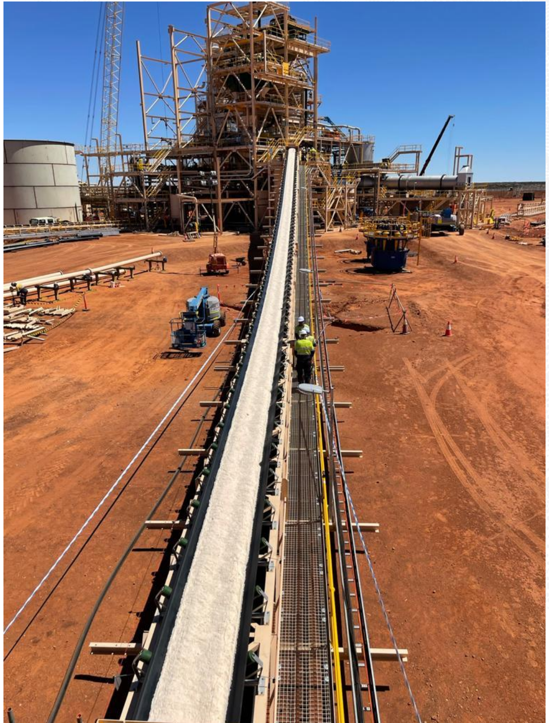
Figure 3: Conveyer CV02 and Process Plant
