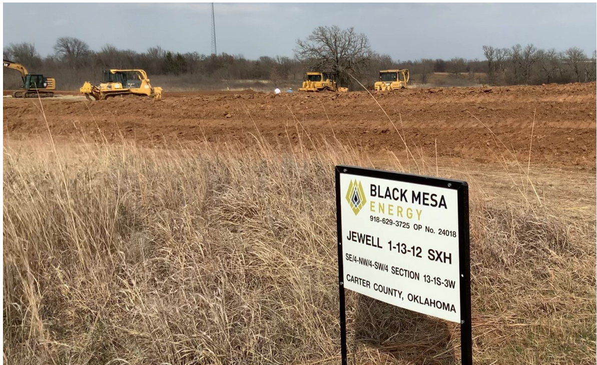
Figure 2. Earth moving equipment on site constructing the Jewell Well pad
