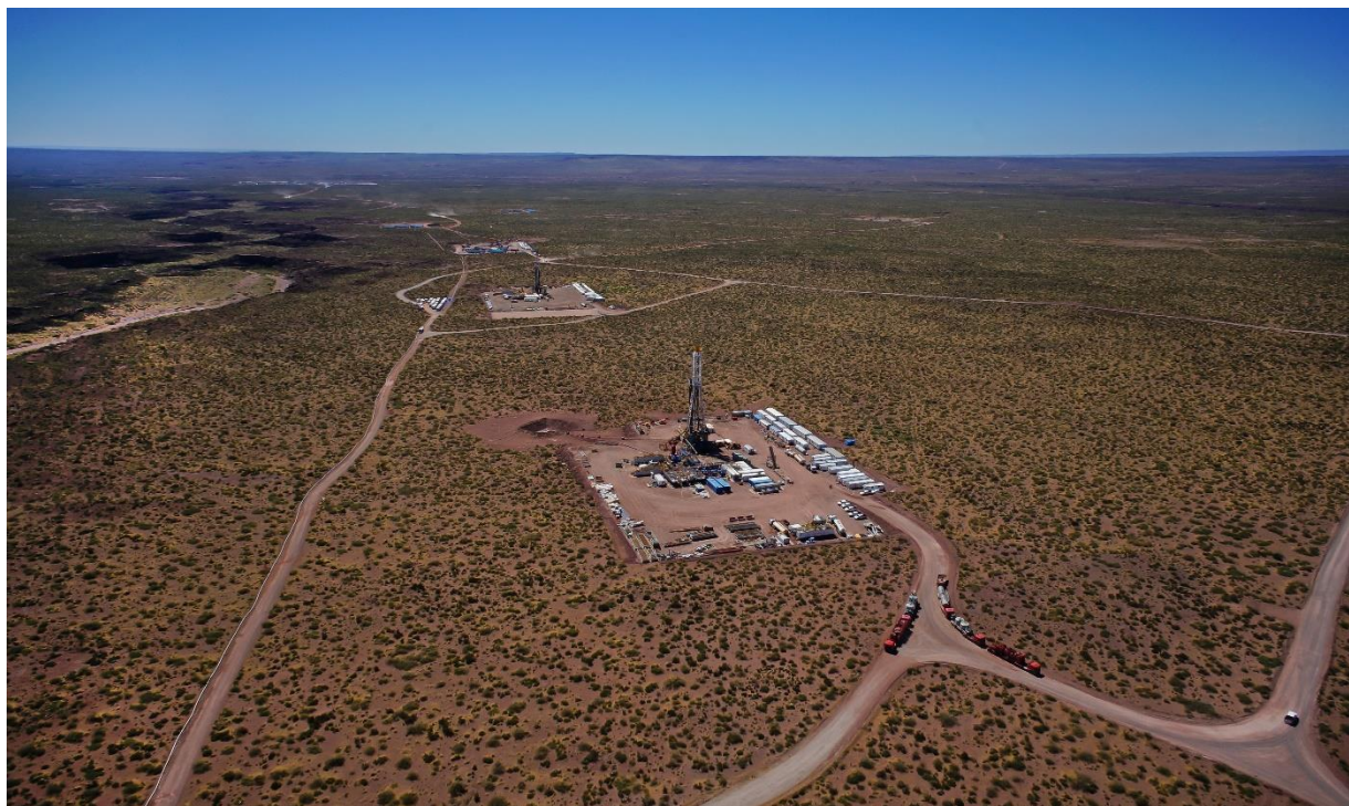
Figure 2. Example of a land based oil and gas drill pad and rig similar to that proposed for the Jewell well.
