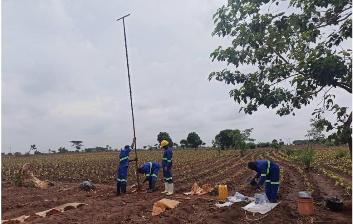
Figure 3. Sovereign’s field team hand-auger drilling at Nsaru.
