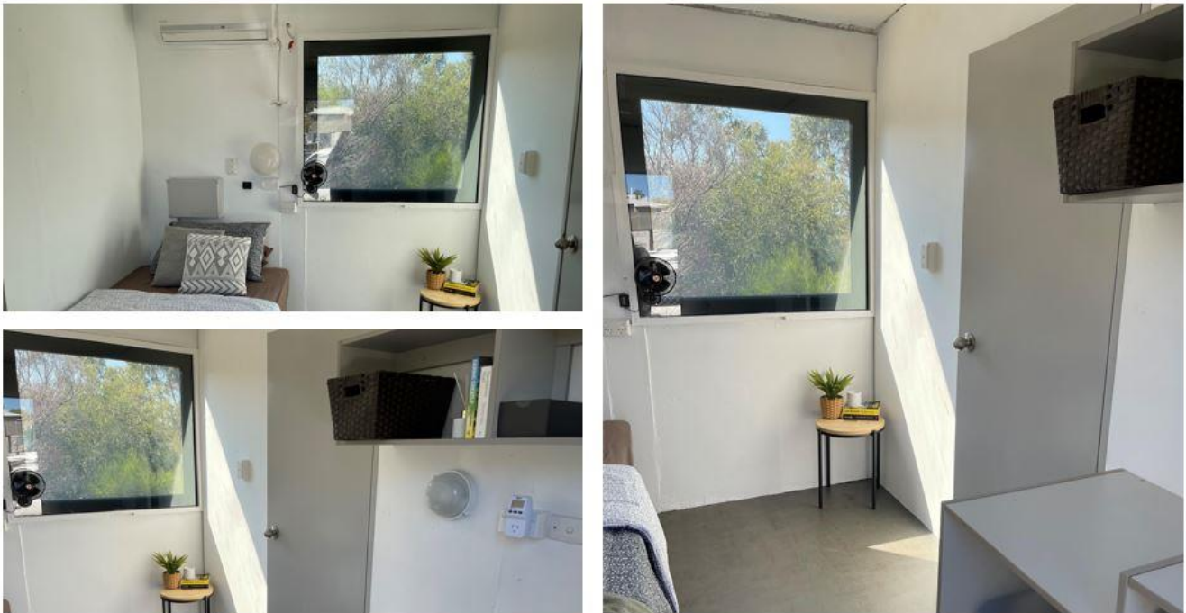
Interior of the ATCO mining hut retrofitted with ClearVue PV IGUs and Mirreco's Hemp panel insulation – view is through the installed IGU panels.
