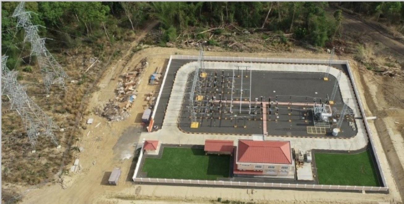
Figure 4 | Electrical Sub-Station, materially complete- ready for commissioning
