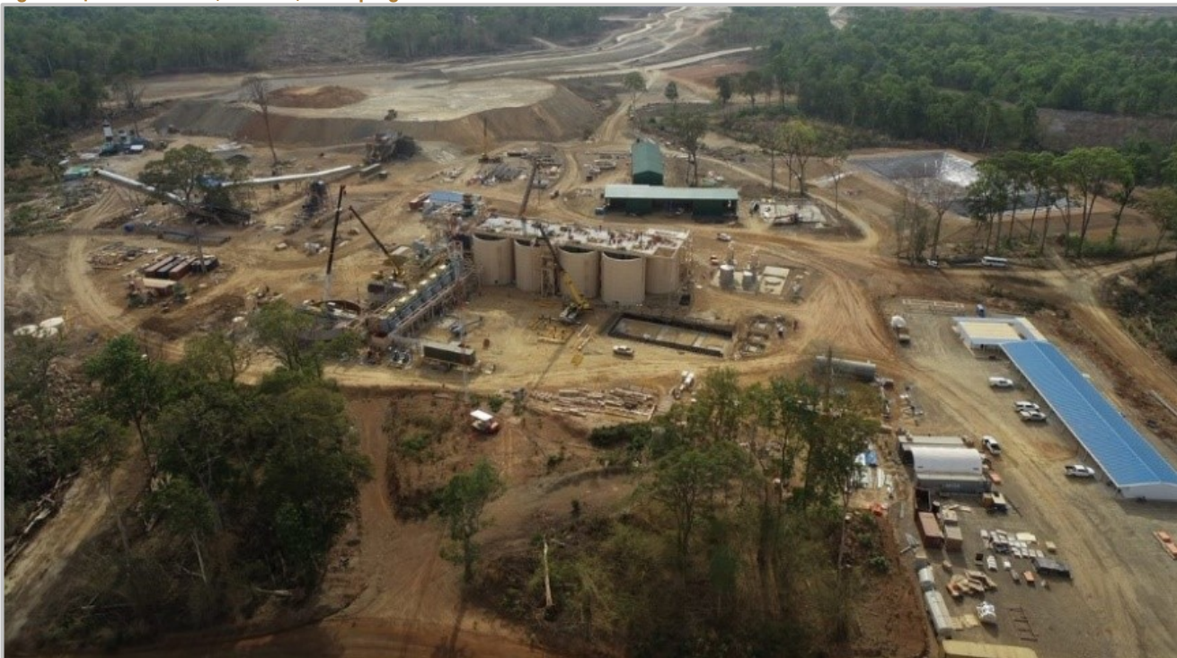
Figure 2 | Process Plant, Crusher, ROM progress
