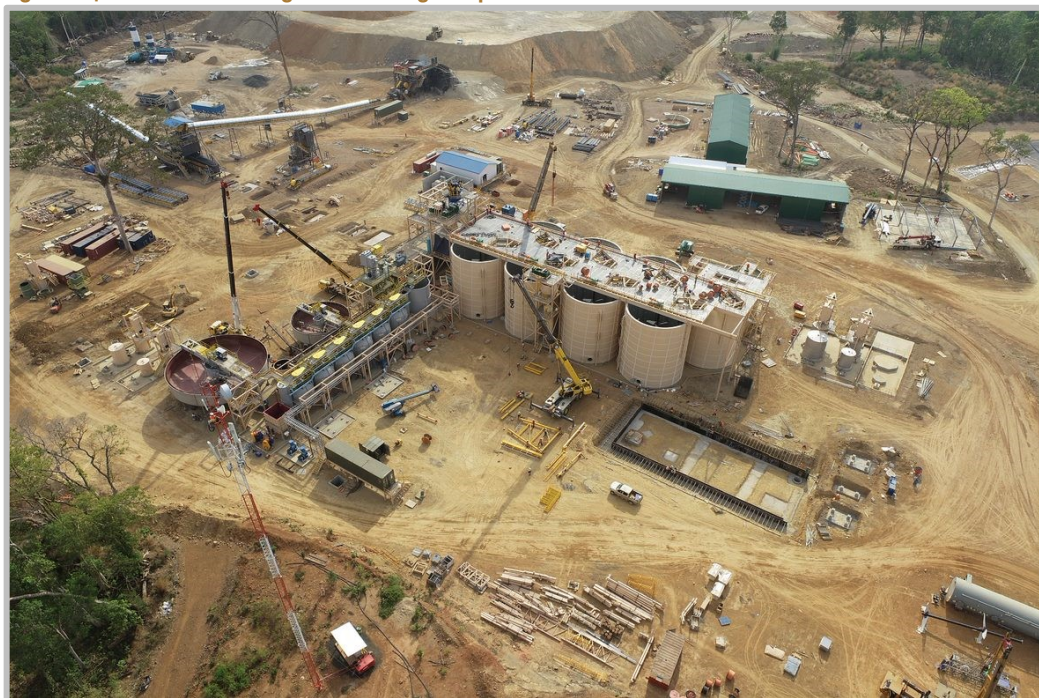
Figure 1 | Process Plant Progress - nearing completion
