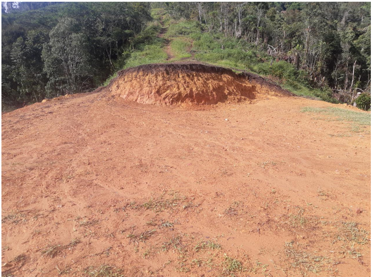
Photo 1: Constructed Drill Pad PDH30A & B Completed and Ready for Drilling.
