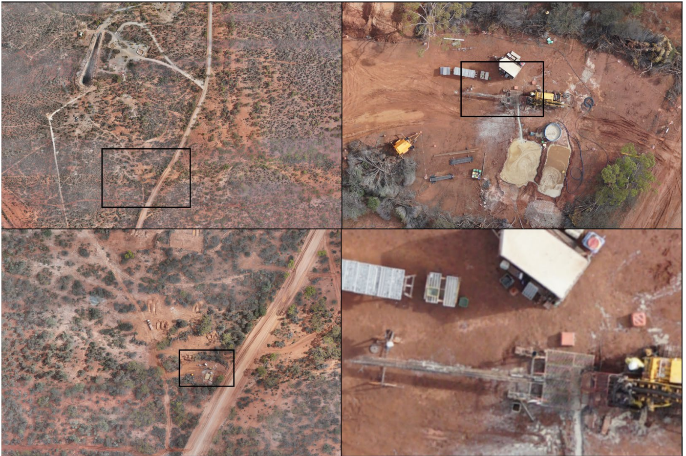
Figure 32; High resolution Wingtra survey providing 1.6 pixels per cm 2 . The images show the available resolution from the aerial survey allowing details to be observed down to core boxes at the drill rig and the driller at the control panel on hole VDD001.
