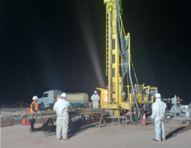
Brine production wellfield drilling
