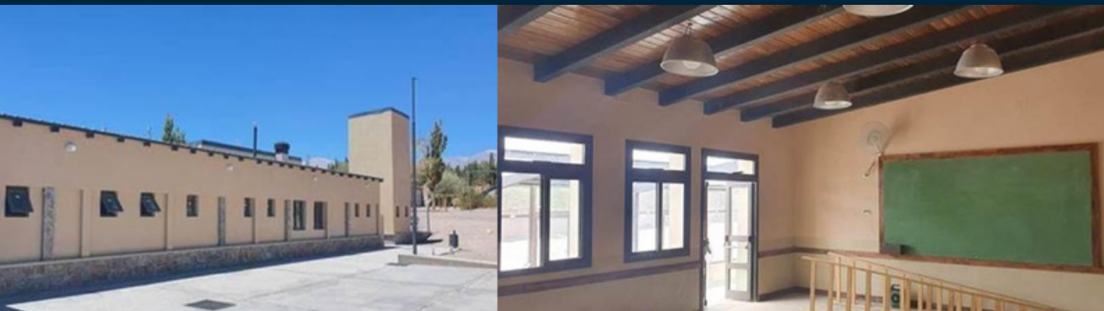
Post reporting period, the construction of the high school in El Peñón village was completed and handed over to the Ministry of Education
