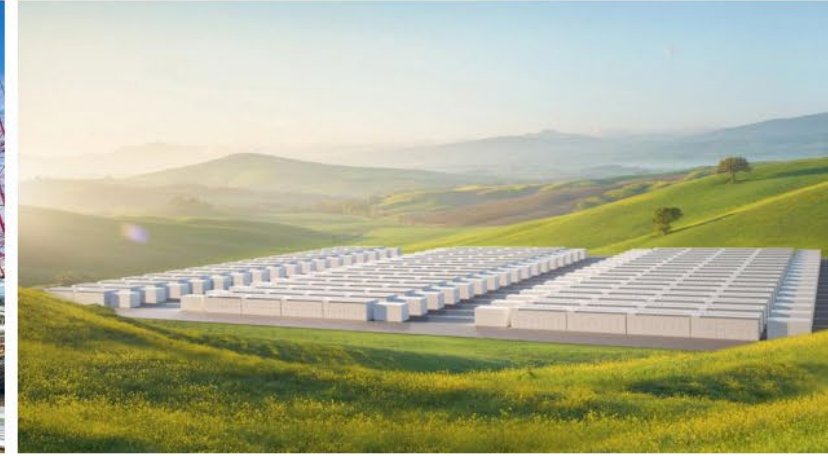
Moss Landing Energy Storage California
