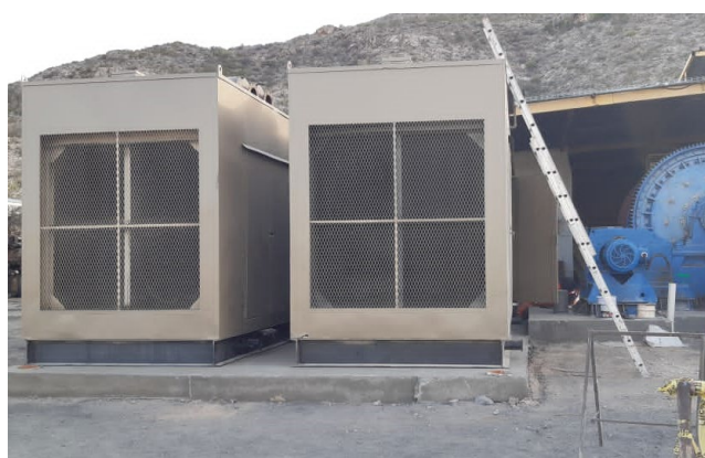
Two 1MW gensets installed 20 March 2021
