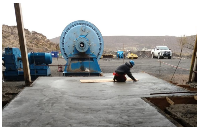
Mill foundations being finalised January 2021
