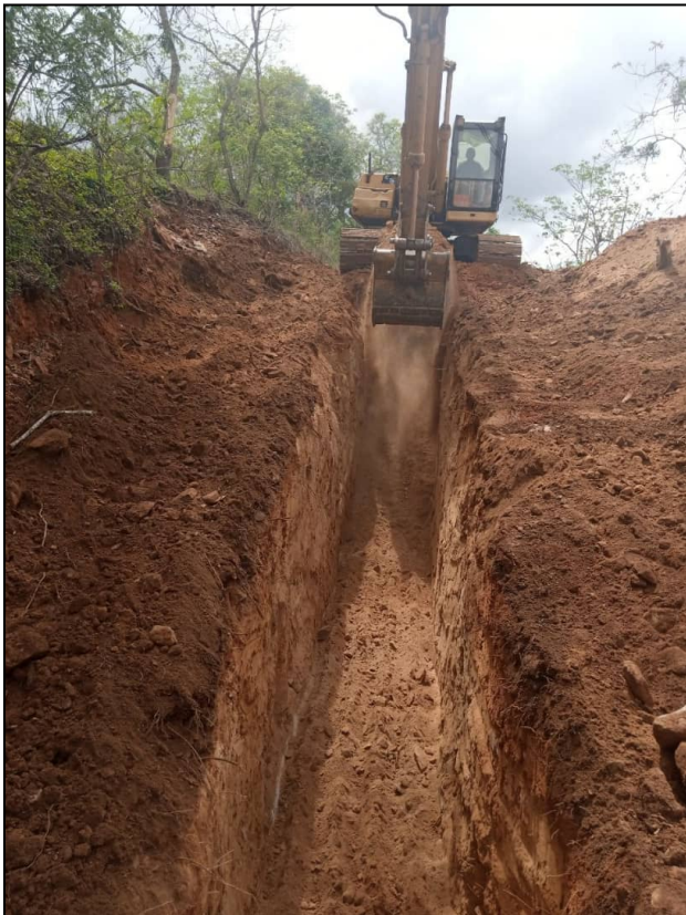
Figure 5 – Trenching begins at the Dragon Target
