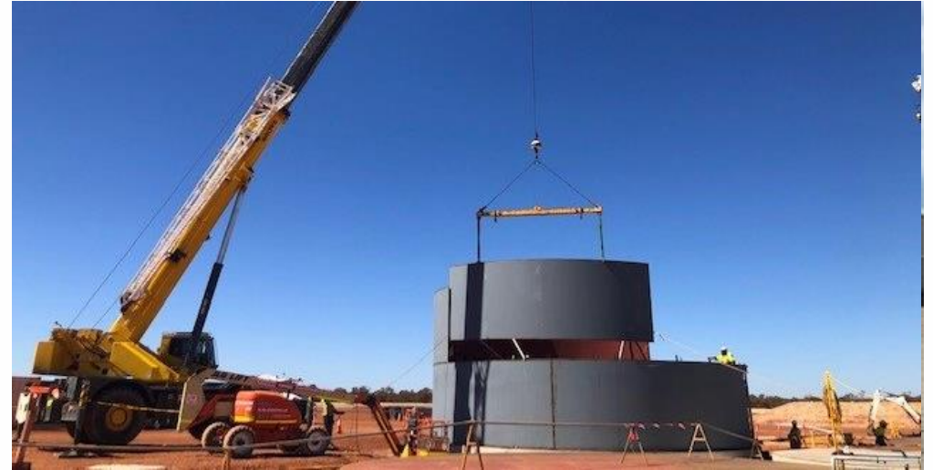
Installation of CIL tanks
