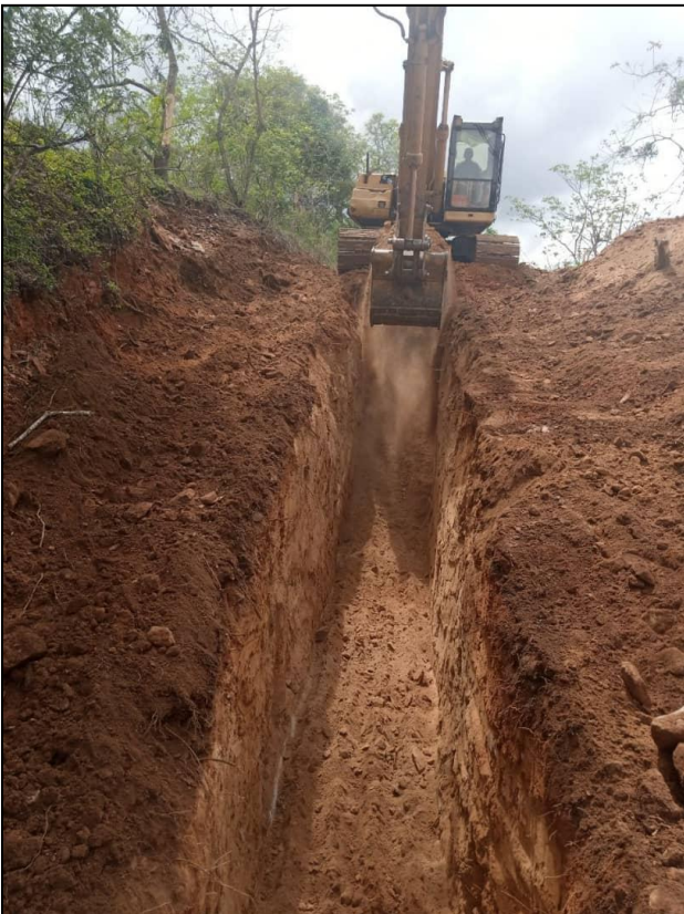
Figure 5 – Trenching begins at the Dragon Target
