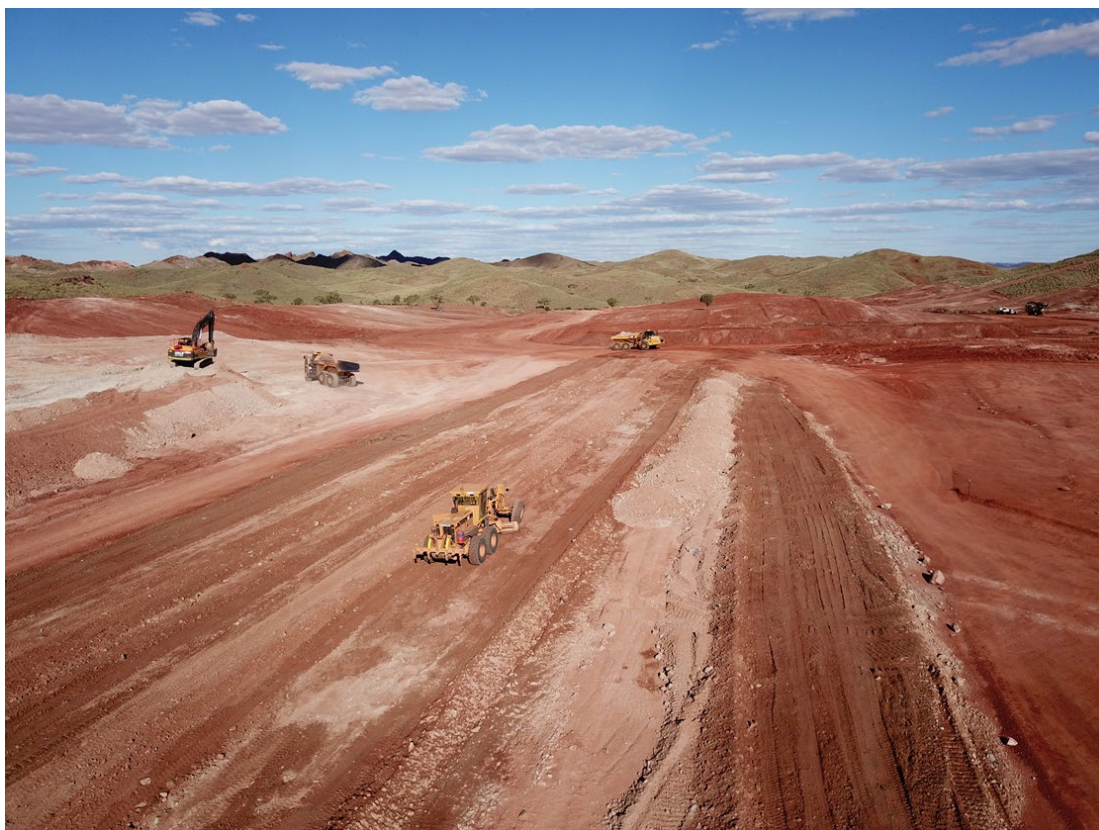
Figure 3: Bulk earthworks at process plant well underway
