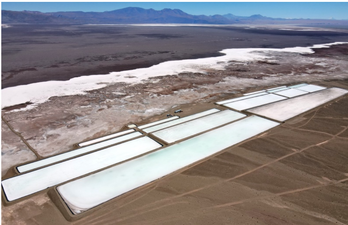
Figure 2. Rincon Lithium Project – 38Ha Operational Evaporation Ponds
