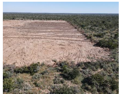
Site camp clearing
