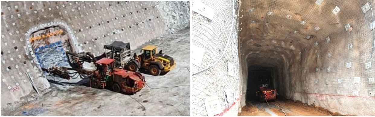
Figure 3: Garden Well South portal establishment and initial development drive.
