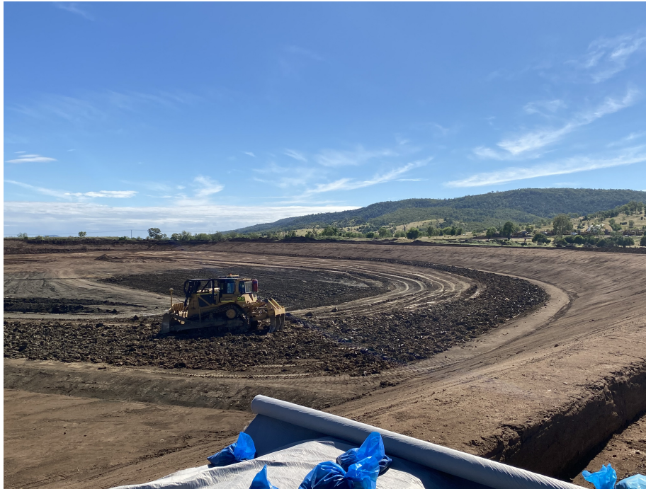
Figure 2 – Cracow TSF No.2 under construction
