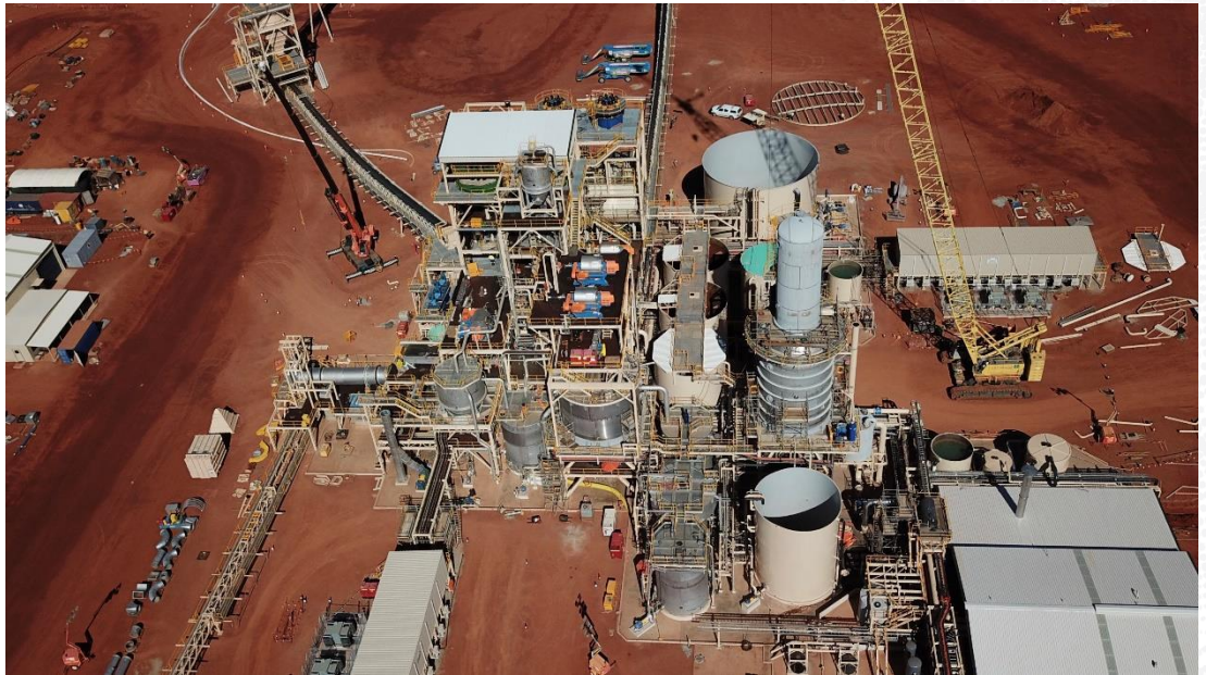
Figure 3: Process Plant aerial view
