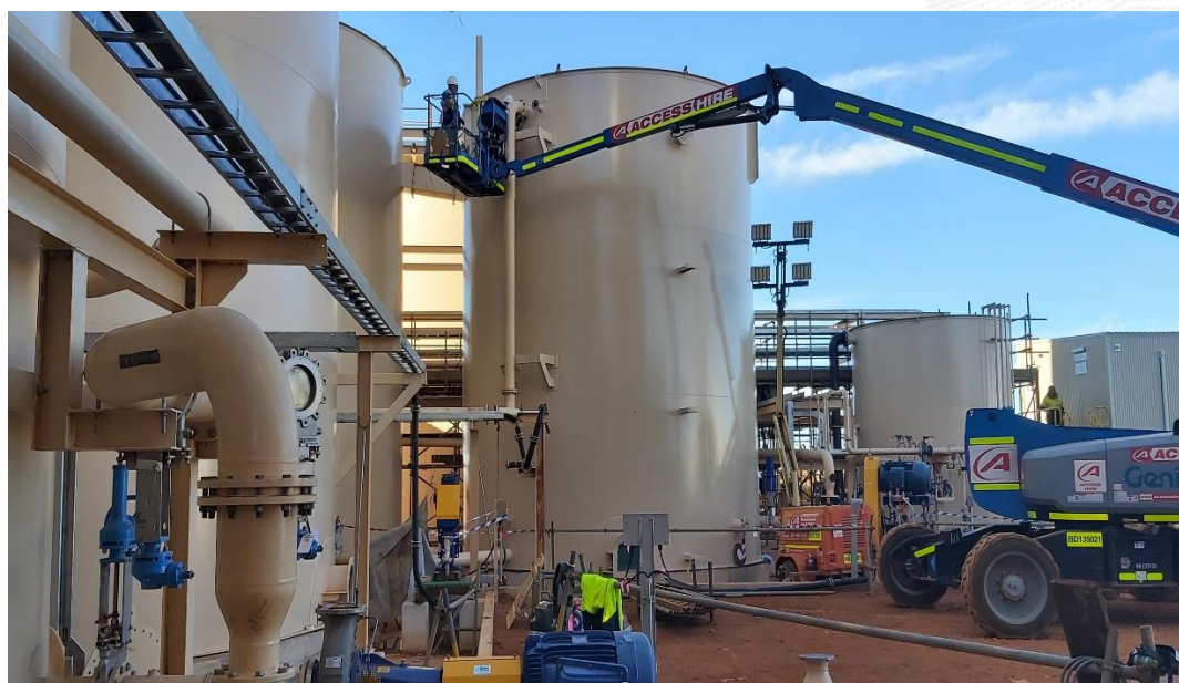
Figure 5: Various tanks/piping completed during the quarter as commissioning activities ramped up
