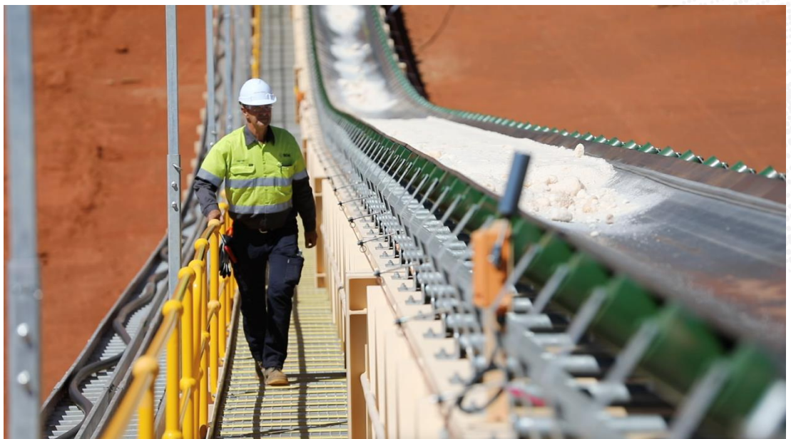
Figure 2: Conveyor CV01 operating with first feed salts
