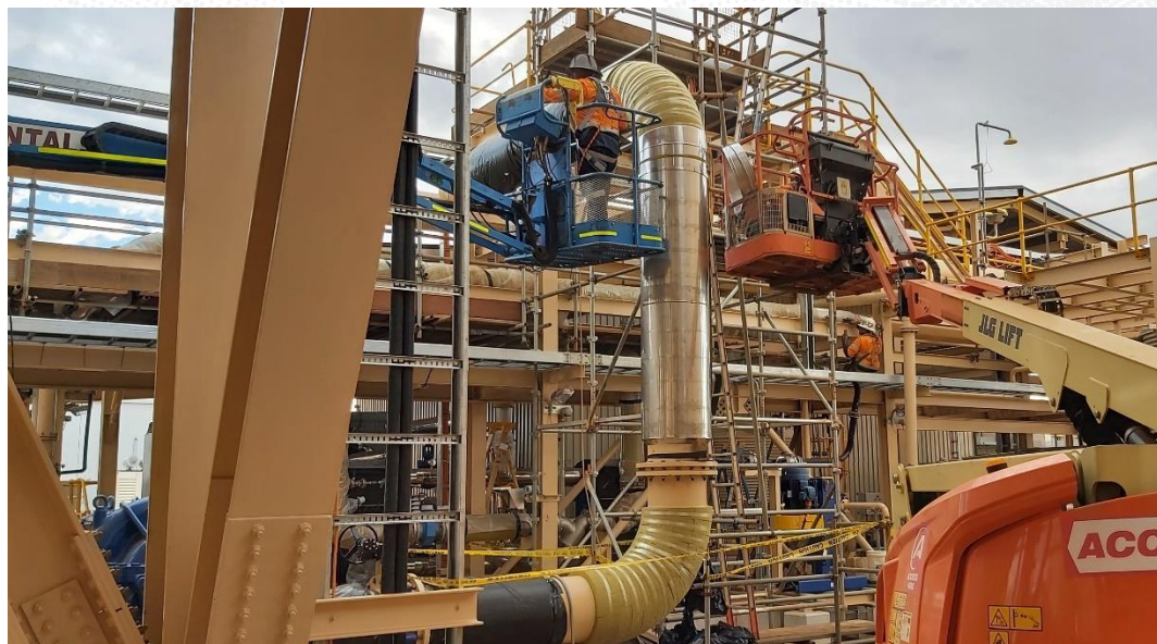
Figure 4: Installing thermal insulation to chilled water pipework
