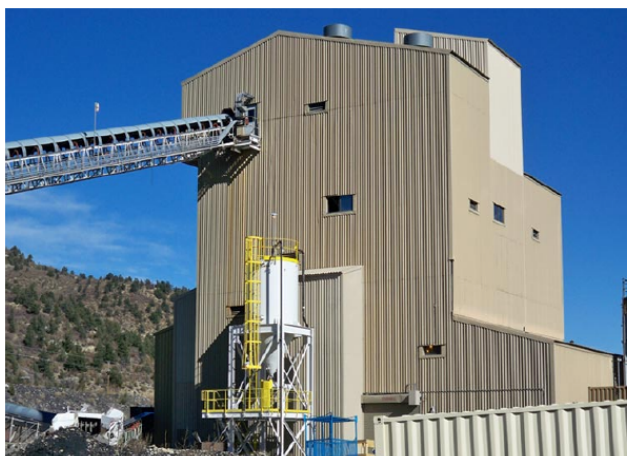
Coal processing and preparation plant
