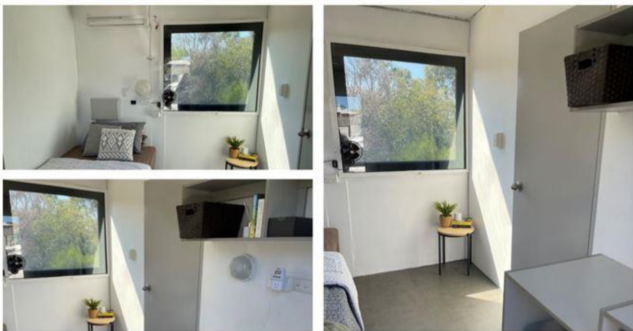
Interior of the ATCO mining hut retrofitted with ClearVue PV IGUs and Mirreco’s Hemp panel insulation – view is through the installed IGU panels.
