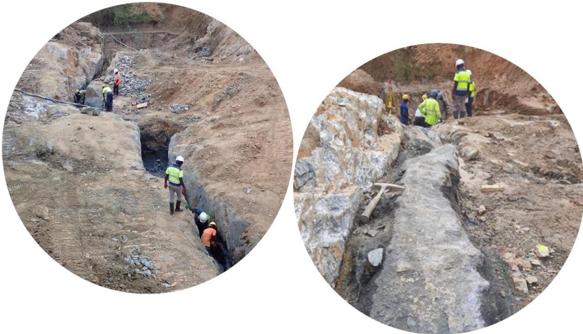
Figure 4: Bulk sampling of the Peyima kimberlite dyke
