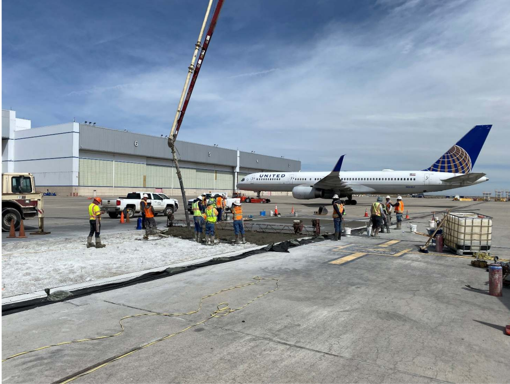
Figure 1 Replacement of first concrete panel on United Airlines maintenance hangar apron.
