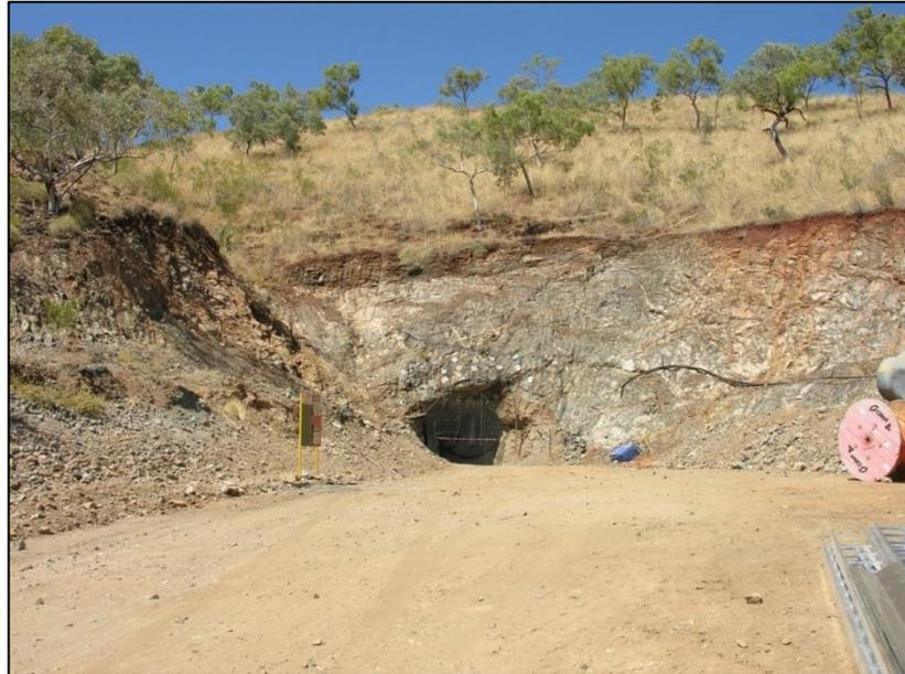
**Figure Three | Exploration Portal and Decline Access**
