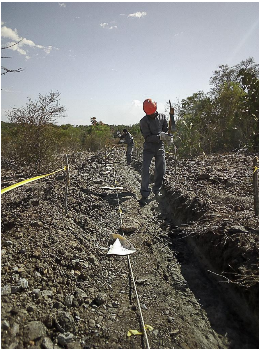
Figure 1 – Trenching continues in the Northwest Razafy Area
