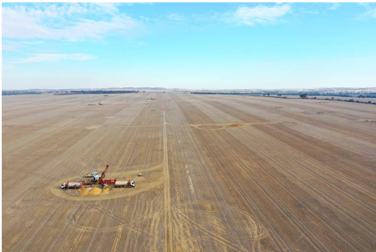
Aerial image showing drill rigs in operation at Bindi
