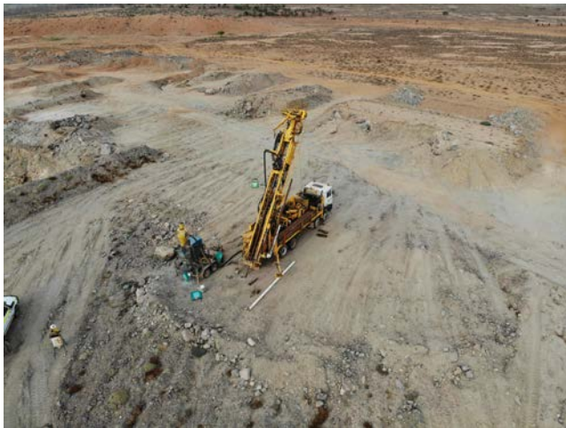
Rig in position for hole 1
