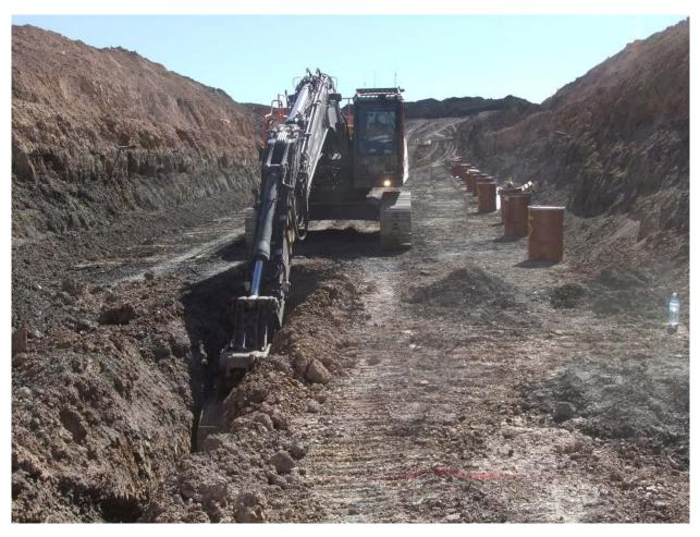
Image 2 | Excavating sampling trench into the heap leach pads
